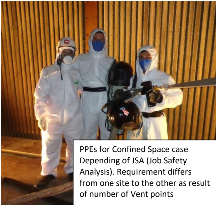
BA system used during the cleaning without impacting the technician movements.
