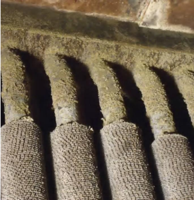
Top & bottom manifold of boiler: Most important part of the boiler
